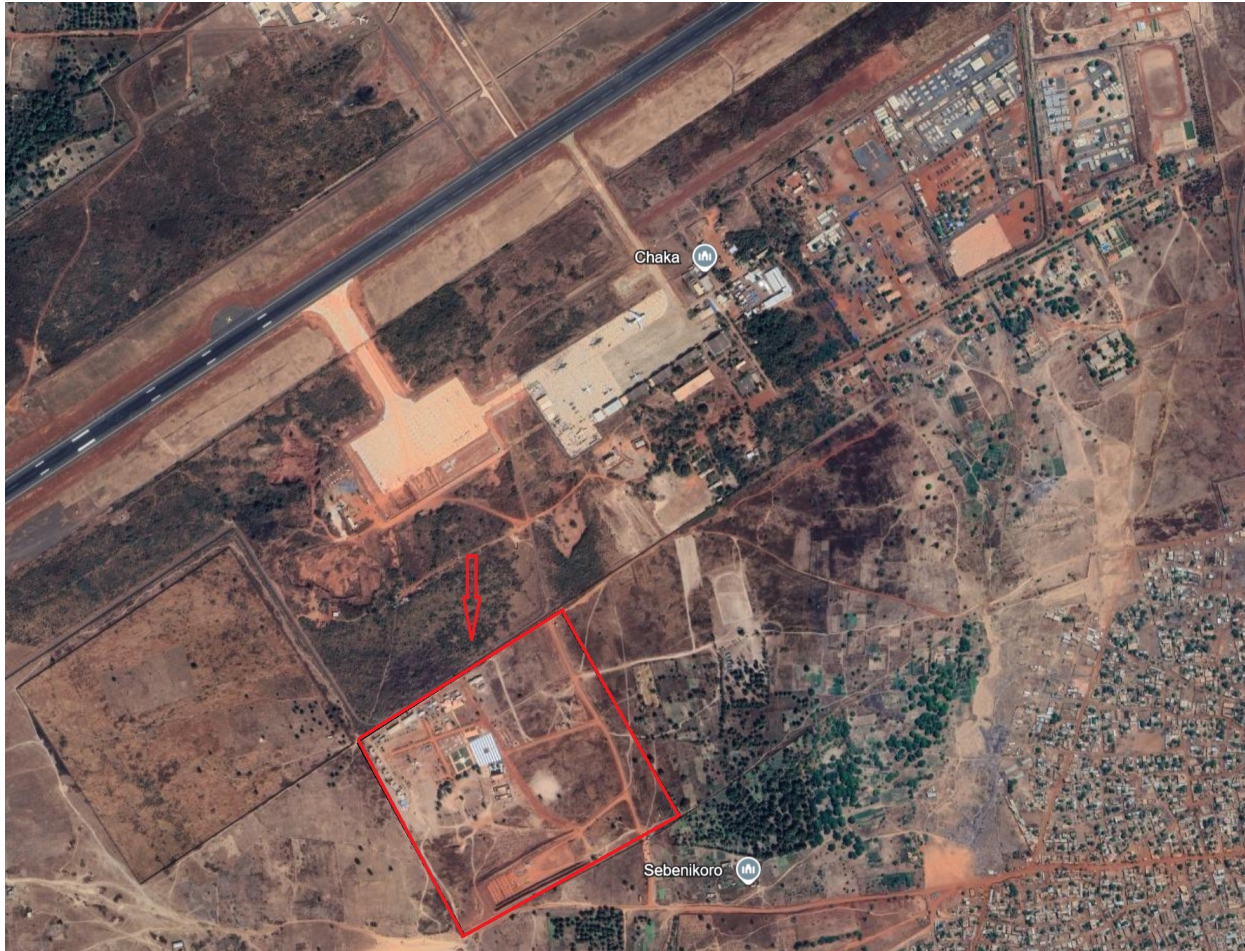
The Russian Africa Corps base adjacent to Modibo Keita International Airport, Bamako, host to the aviation and air defence assets discussed in this note.
